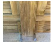
Mi-T° Post Cover Boards can be used to cover the rear side of a galvanised Mi-T° post.
